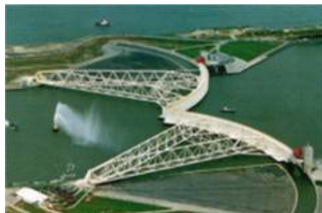
The most recent and final addition to the Delta works: the Maesland flood gates (scale: put upright, each gate is as high as the Eiffel tower)
